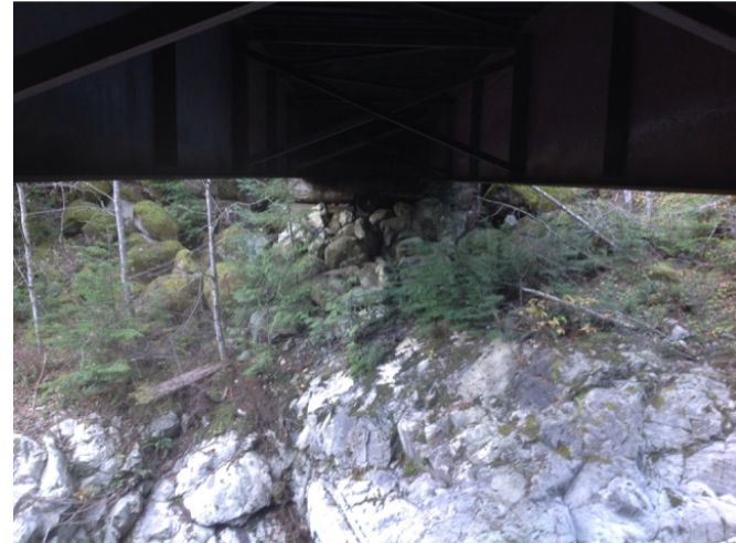
Right Bank Abutment when facing downstream
