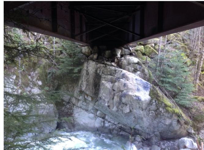
Left Bank Abutment when facing downstream
